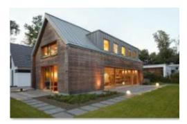
The roof was clad over an area of 180 m<sup>2</sup> with RHEINZINK-prePATINA blue-grey in the angled standing seam system, the timber façade is made of Douglas fir.
