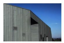
The panels of different widths (300, 400 and 500 millimetres) divide the façade vertically. The installer emphasised building recesses by installing them horizontally.
