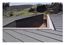
The lower roof termination is formed by an internal rain gutter. The covering of the gutters also serves as the upper finish of the façade cladding.
